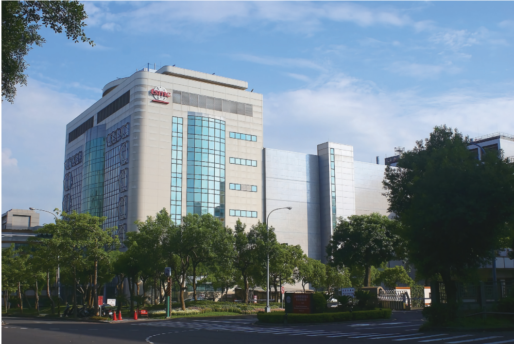
Figure 2. TSMC, Fab 5 Building, Hsinchu Science Park, Taiwan
