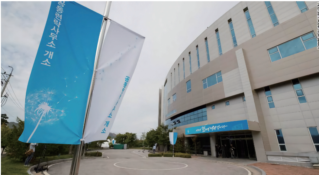
Figure 4. The Joint Liaison Office in Kaesong Industrial Complex
